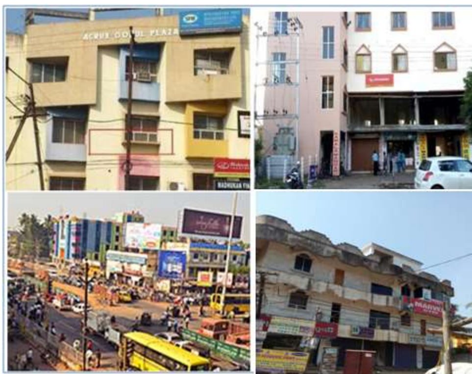
Figure 3-5: Different types of commercial buildings/centers
