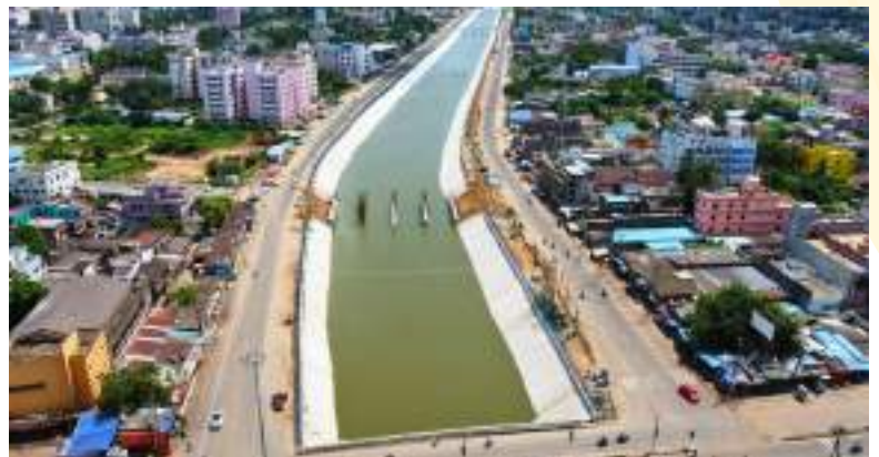
The ongoing Taladanda Canal transformation under 5T program is poised to become the new face of Cuttack.
